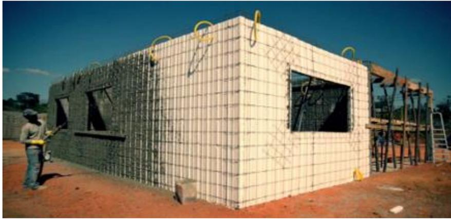
Figure 05: Application of microcement with equipment
